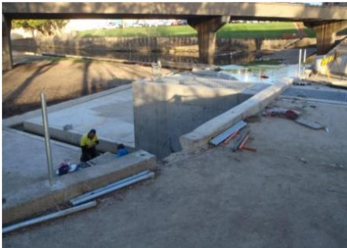
The photos at left and below were taken in early August and show the lock nearing completion. In fact, the contractor can be seen fine tuning the electrics and only the temporary bunding need be removed to make the fishway operational. The lock controller is set to cycle through the lift process every 20 minutes – a lot better than the 190 odd years that fish have been waiting since the last free access was available!
