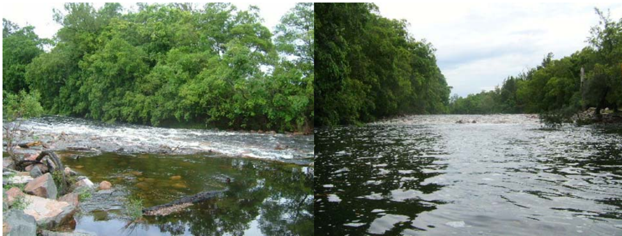
Fishway looking downstream
